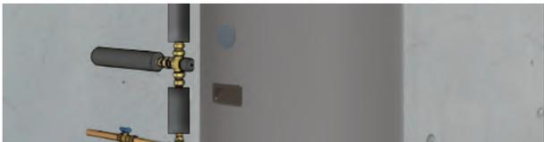
Connect cold water pipe and hot water pipe to the tempering valve.
